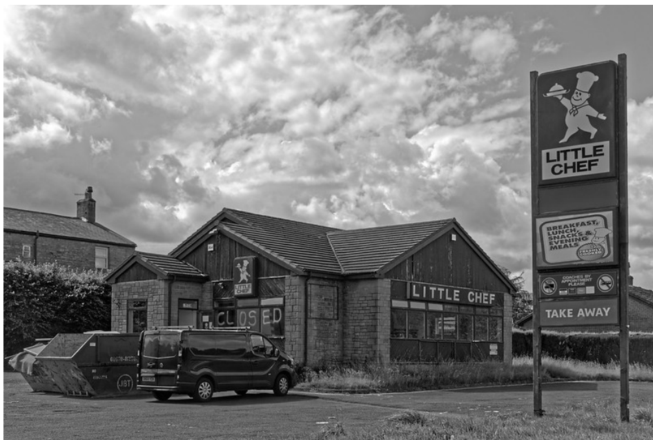
Figure 16 Infrastructure around Haltwhistle connects the town but lack of investment can create problems. Source: "Little left of Little Chef, A69, Nr Haltwhistle" by A C Skinner (CC BY-NC-ND 2.0.)
