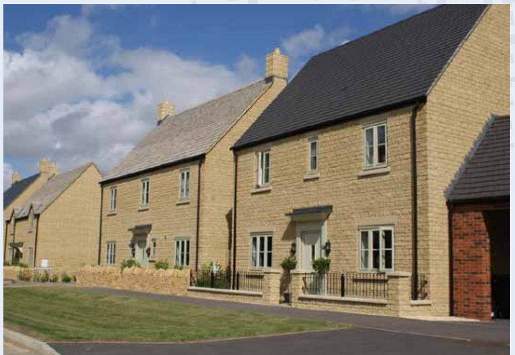
High quality new homes, built from the local Cotswold stone.
