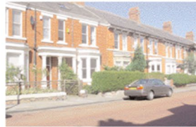
Regular - almost a 'grid iron' - layout of blocks in a suburban context. Jesmond, Newcastle
