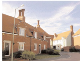
An irregular block structure providing an 'organic' and intimate character. Thorley Lane, Bishops Stortford
