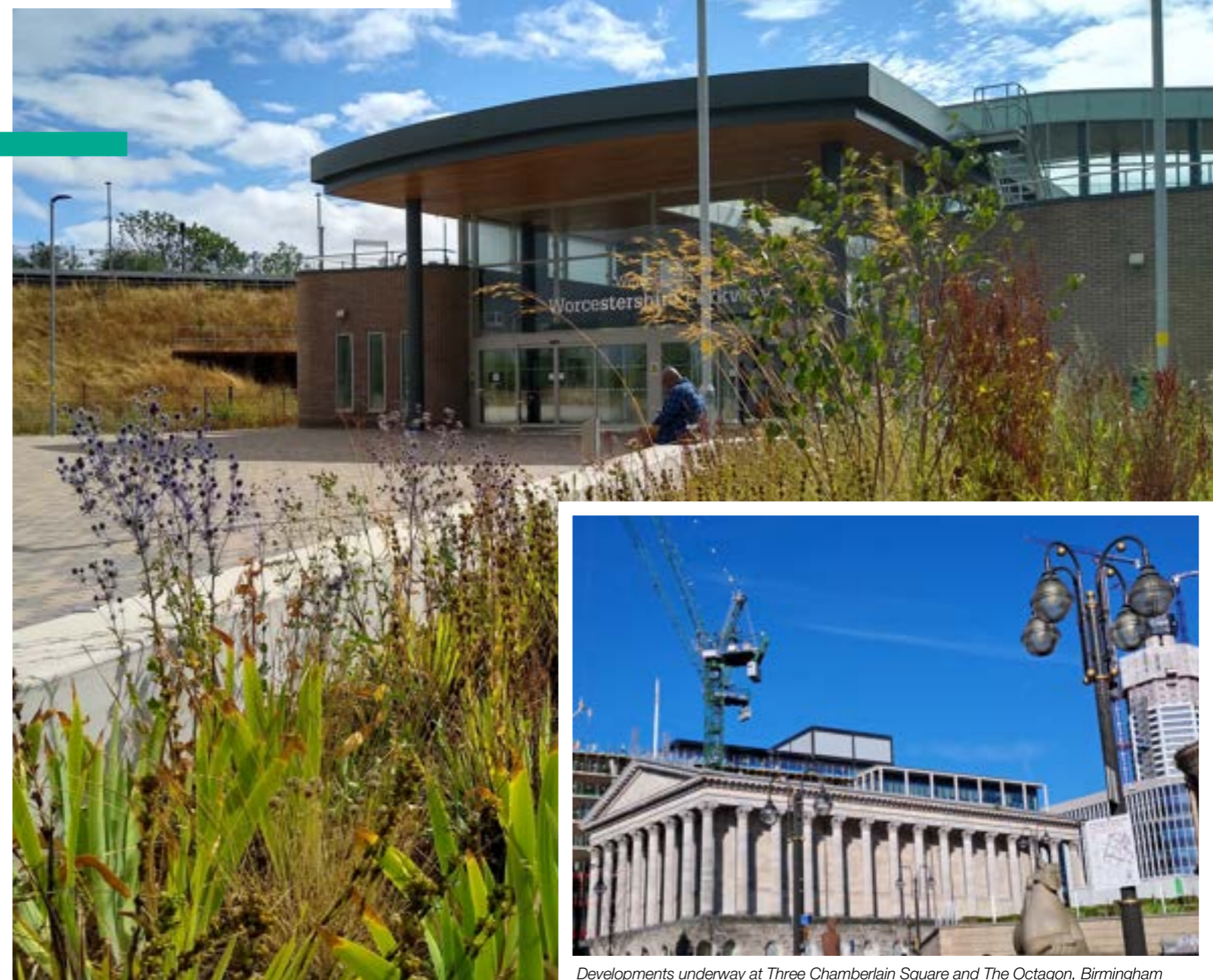
Developments underway at Three Chamberlain Square and The Octagon, Birmingham
