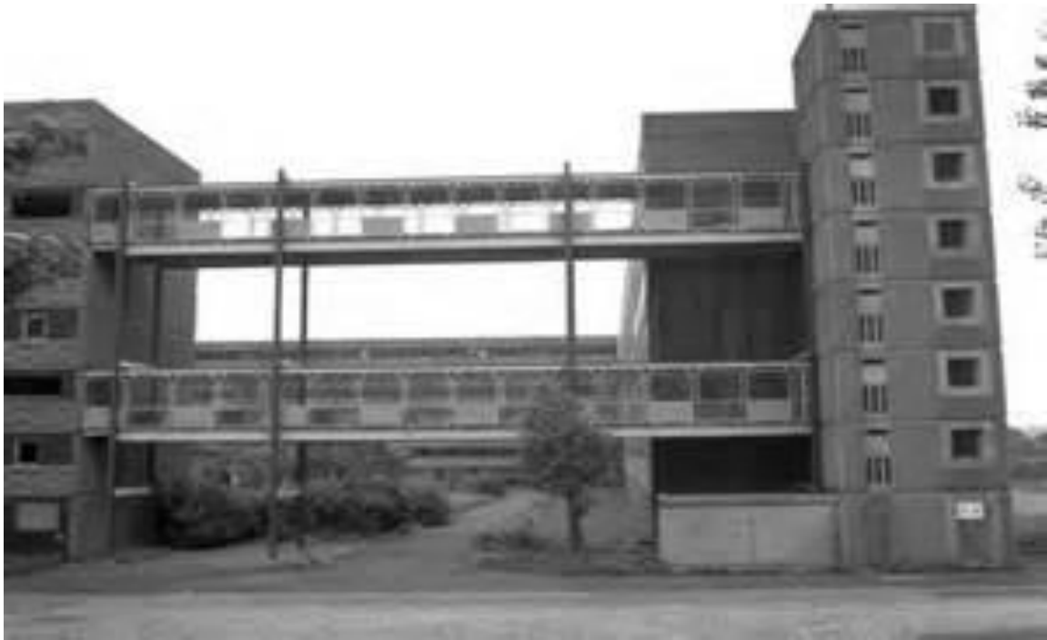
Pic. 2. The then derelict Hutcheson E residential block, Gorbals
